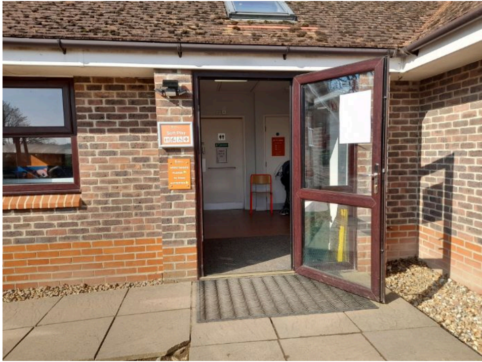
Access to the Soft Play building.
