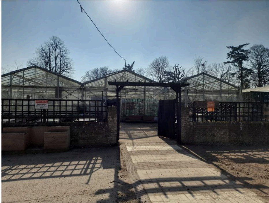
Entrance into the Greenhouse.
