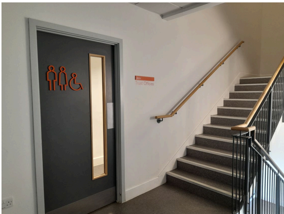
Access to toilets from the Quarry Café. These doors are not automatic, and push inwards.
