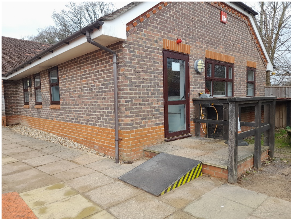
Ramp to exit 3-5 years Soft Play room (shown above).
