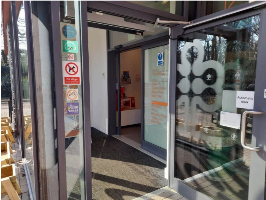
Entrance door into the Gift Shop / Reception area.
